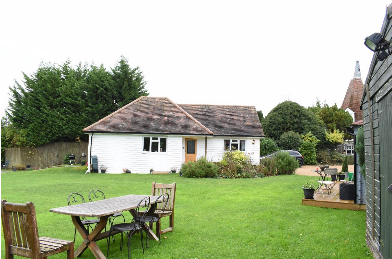
Plate 9: View across the PDA towards the annexe (facing SE).
