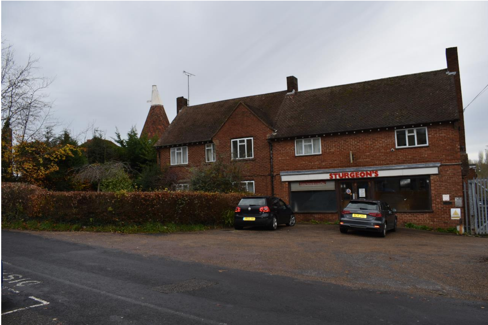
Plate 11: View of Sturgeon's, which will eventually provide access to the PDA (facing N)
