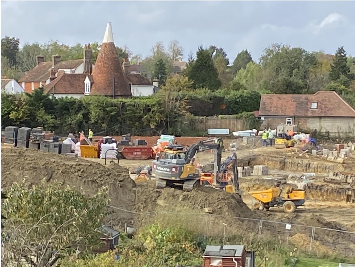
Plate 17: Construction underway at the adjacent Sturgeons site (facing NW)
